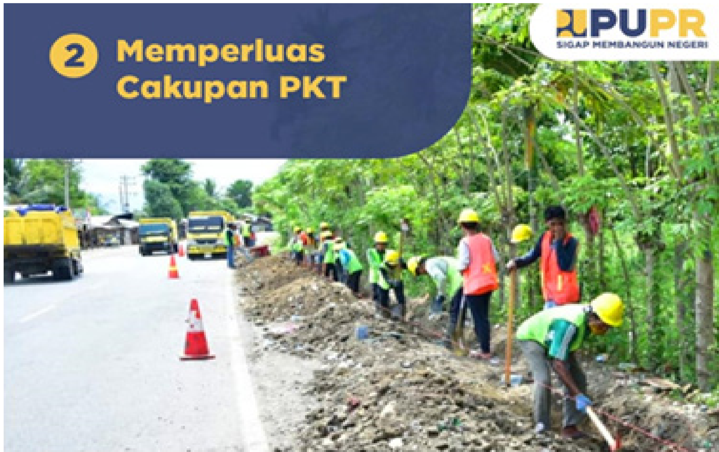
Figure 1: Examples of drainage revitalization and bridge painting on road preservation projects Source: www.pu.go.id .
